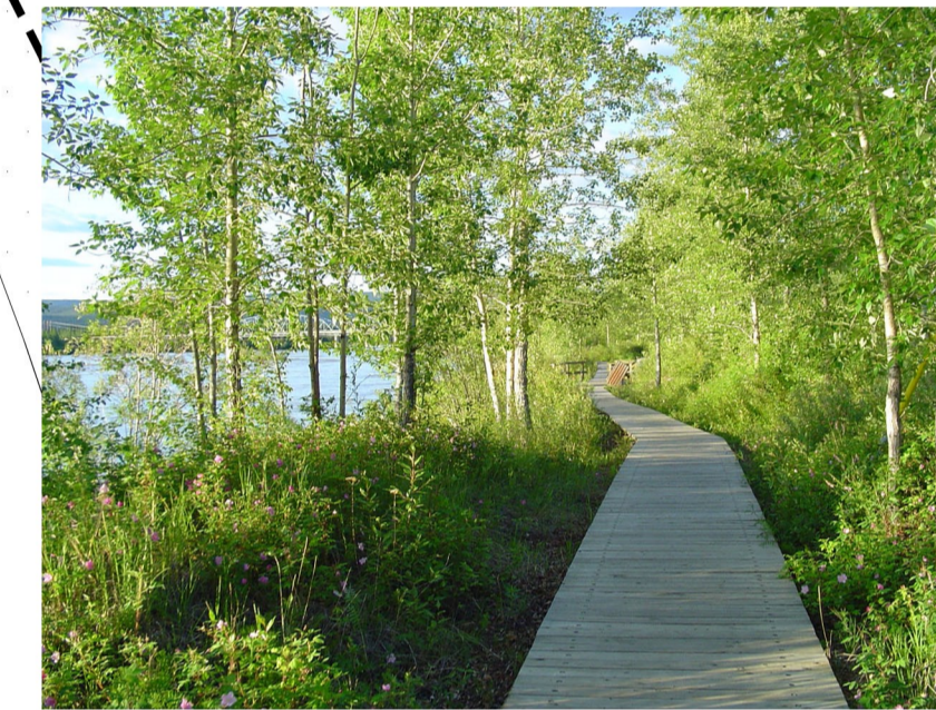
Timber Walk Platform
